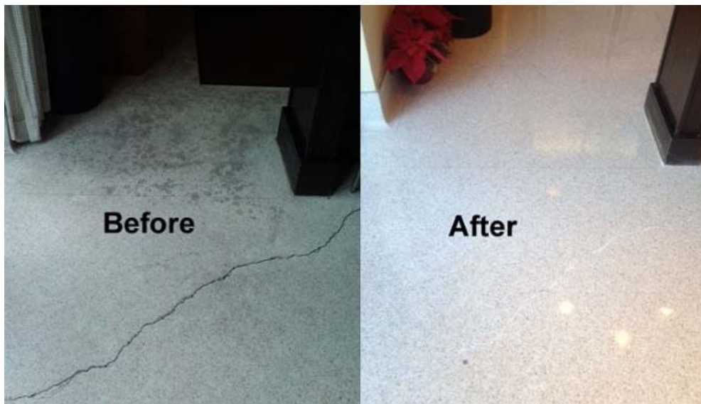
One of Jacqueline's favorite before and after photos of terrazzo floor restoration
