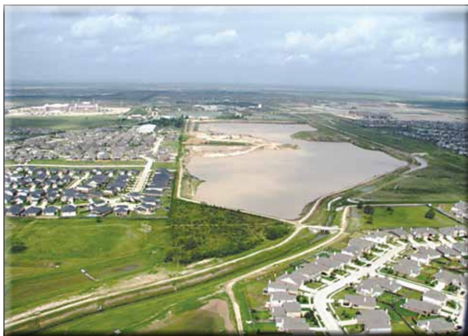
An aerial view of the Horsepen Creek stormwater detention basin
